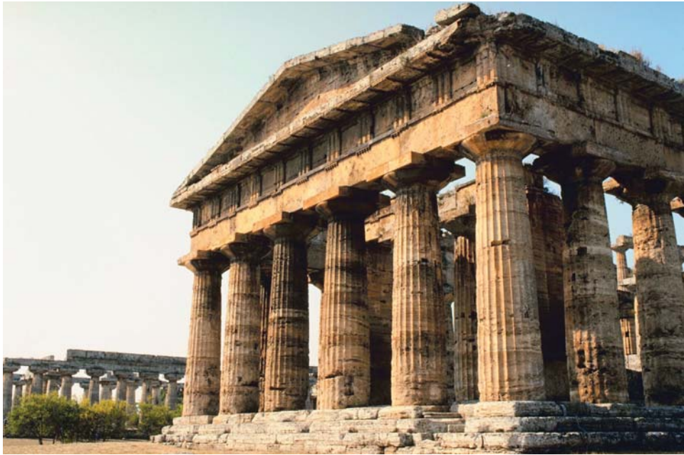
Hera’s temple in Paestum in southern Italy dates from the fifth century BCE. The Doric-styled temple features 36 fluted columns.
